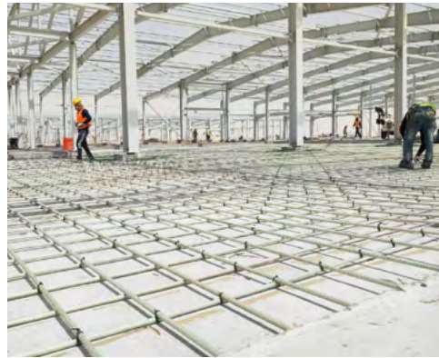
Industrial Slab & Warehouses
